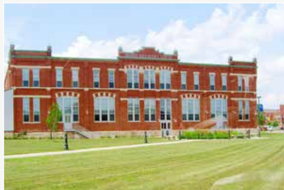
Gund Brewery Lofts (La Crosse, WI, 2007). The 123,000 SF, 86-unit apartment complex is located adjacent to the Gundersen Lutheran Medical Center. It contains a mix of unit types, as well as a mix of market-rate and subsidized rental units. The project has revitalized the 1903 bottling plant that is located on South Avenue. Beyond the adaptive reuse, sustainable features of the project include a solar hot-water system, low-e windows, above-code insulation and the use of native landscaping.
