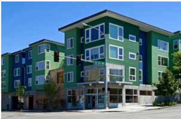
West Seattle Community Resource Center (Seattle, WA, 2007, $8.1M) combines 34 apartments for homeless and low income families, and offices for agencies / non-profits serving low income residents including the West Seattle Food Bank. The LEED® Silver certified, 50,000 SF project was built on a brownfield site on a major urban corridor. It has a central courtyard with children’s play space. The building is owned by the Delridge Neighborhoods Development Association and the West Seattle Food Bank.
