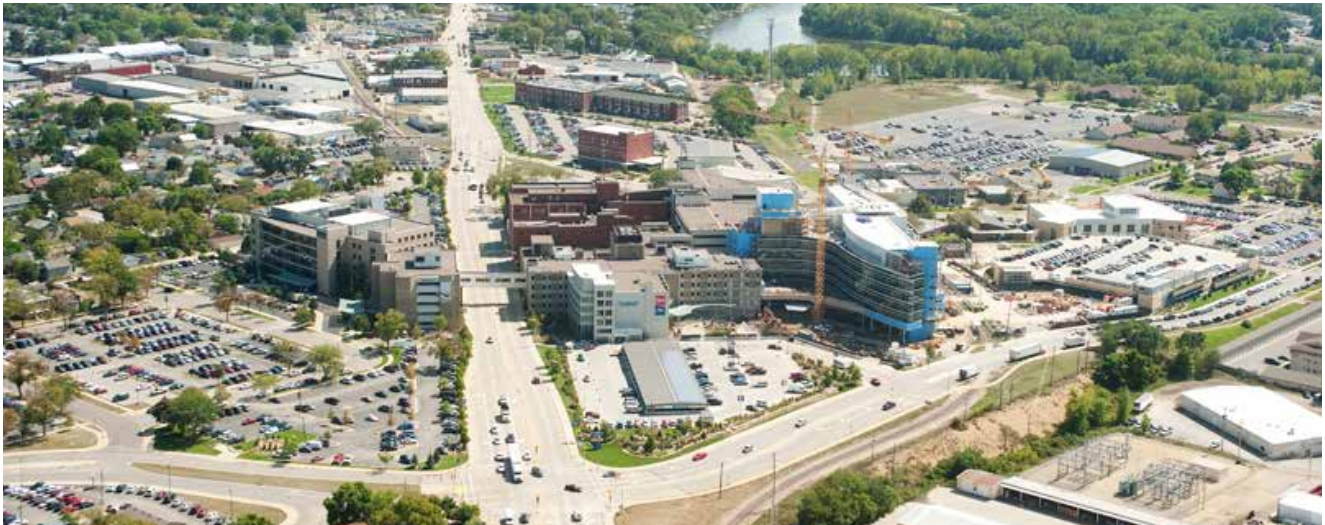
Bird's Eye View of the Gundersen Lutheran Medical Center (2012) showing the new hospital building under construction.
