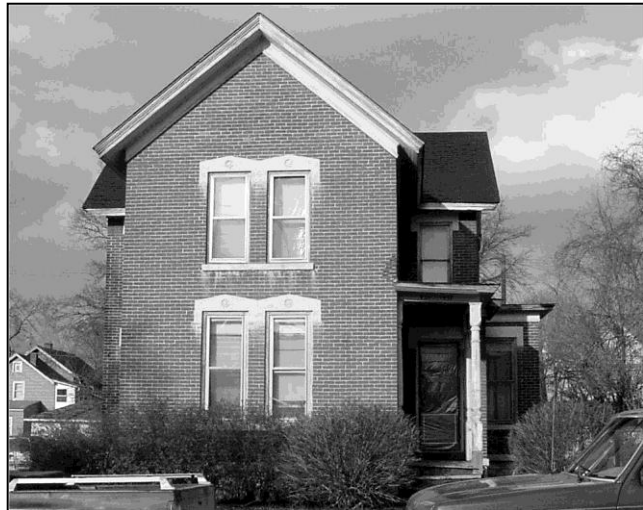
Recently Demolished Home. 1000 Block Ferry St.
