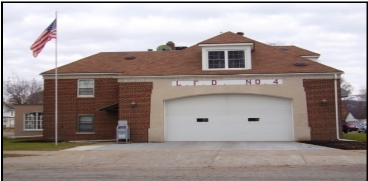
Station 4 at 906 Gillette Street – built in 1941 (North District)
