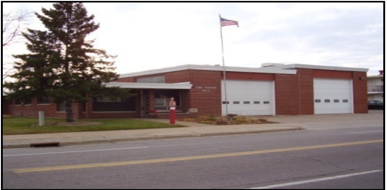
Station 2 at 626 Monitor Street – built in 1957 (North District)
