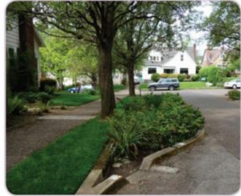
T3 - Vegetative Purification Bed - Portland, OR
